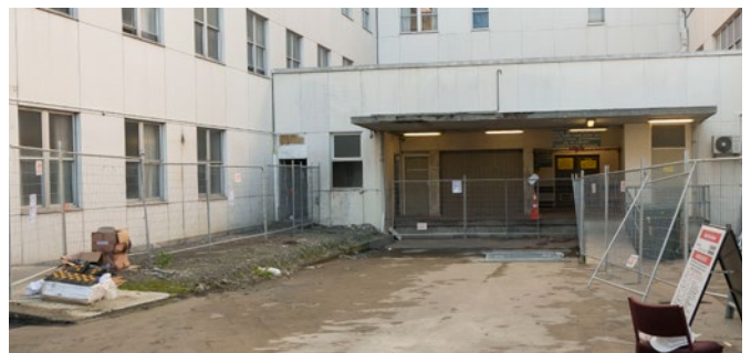
The new temporary clean dock at Christchurch Hospital
