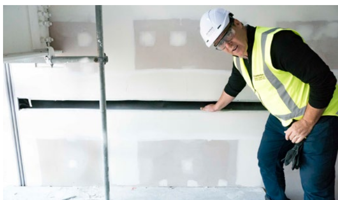
Rob Ojala, Clinical Lead for the Facilities Development Project, shows the seismic gap between levels that is among several seismic engineered features of the building
