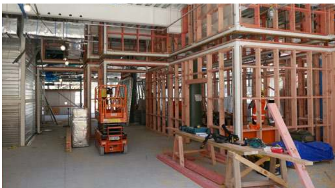
Work on the ground floor docks on the Antigua St side of the building
