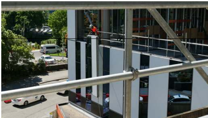
Installing the glass window panels. Currently they are going up at the rate of around 15 a day
